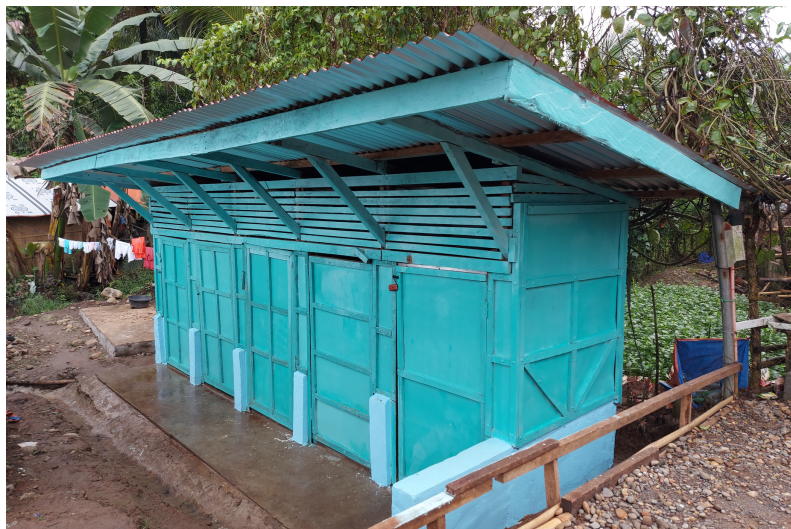
During the needs assessment the lack of sufficient WASH facilities like latrines and handwashing stations was one of the pressing concerns expressed by the community. These structures were also built in consideration of inclusivity and ease of use by vulnerable community members, such as women, persons with disabilities, and older persons.
