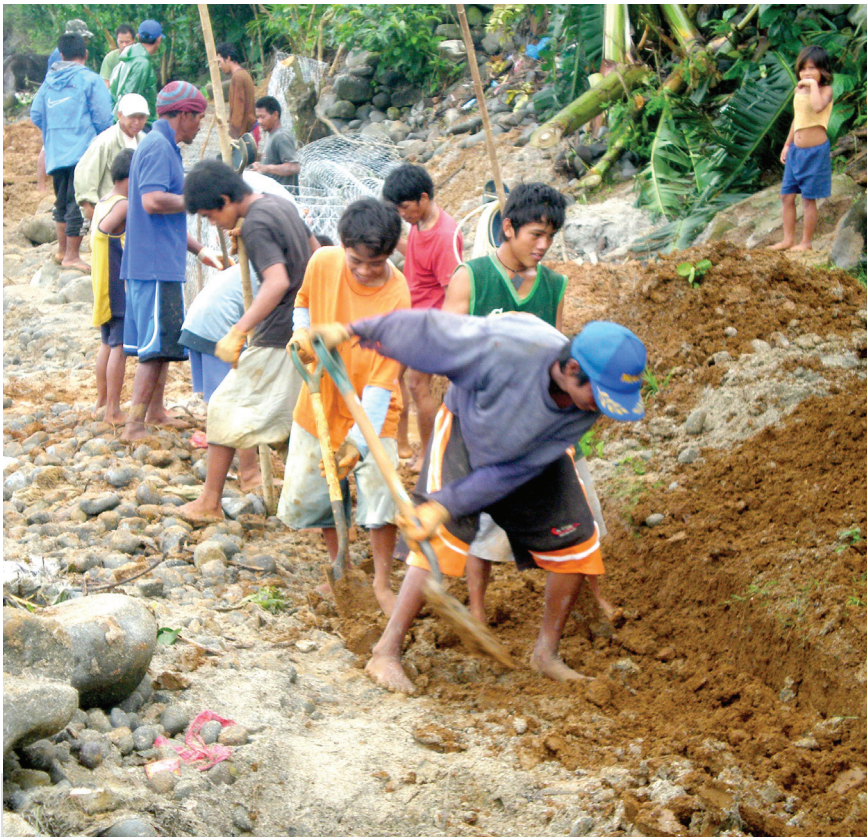
“Rabuz” during installation of Gabion in Bgy. Cagsao in Calabanga
