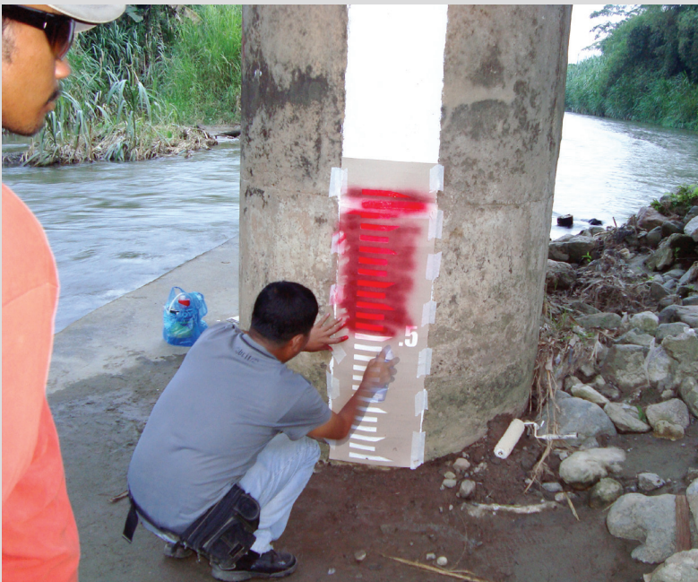
Installation of water-level gauge in Maragusan, Compostela Valley
