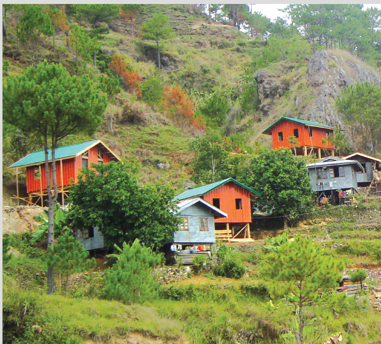
Fifty households from landslide-prone areas in Dalican, Bontoc, now own new homes (in orange) constructed thru "ob-obbo."
